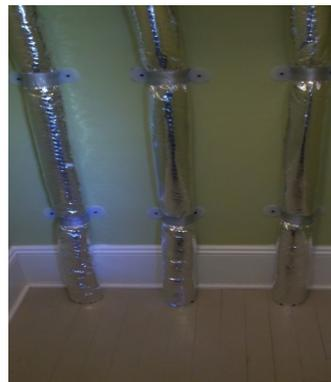
Above: Unico supply ducts running through an interior closet.
